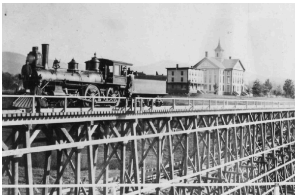
Leased 4-4-0 in use on the big trestle during construction (c1897)
