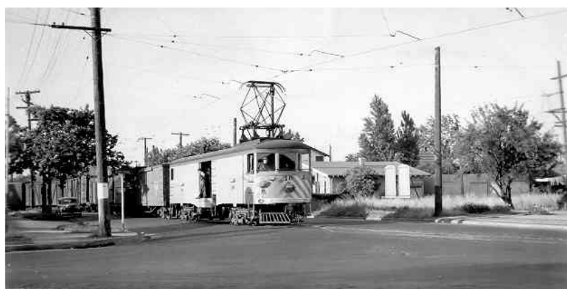
No.#10 - Freight Motor - Cincinnati Car Co. (1930) Acquired Second Hand in 1938 with two other similar units (Nos. # 8 & 9)
