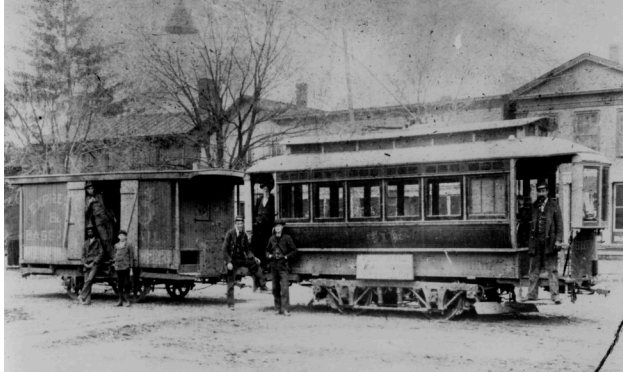
Early electric car and trailer operated by the second iteration of the electric line - The Consolidated Electric Railway - (c.1899) Likely one of four vestibule cars delivered by the Lamokin Car Works to a predecessor line
