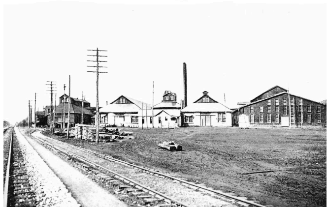
Jewett Car Company manufacturing plant located in Newark from 1904 until 1919.
