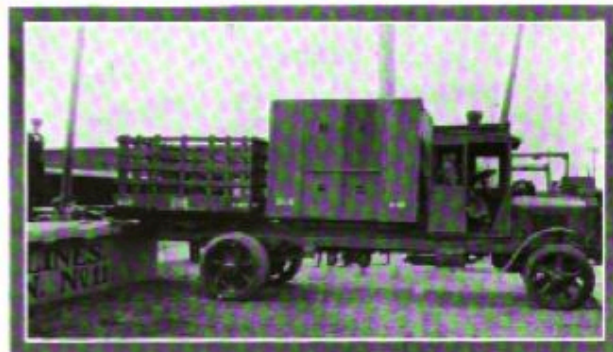
Unloading Containers from Motor Truck to Platform. Note Runway and Wheel Car Under Containers. Detroit
