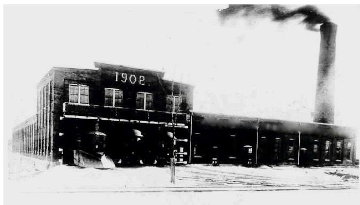
Combination carhouse and power station building
