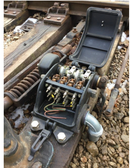
Above: Signal set up on north spring switch. DD
