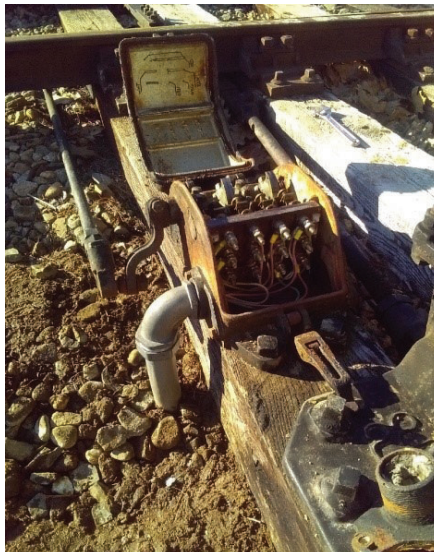
Above: Equipment must be precisely placed. DD
