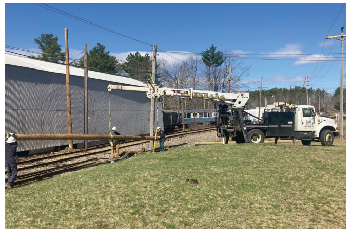
Right Upper and Lower: Two views of Private Power Services replacing deteriorated poles on the main line next to Riverside Carhouse. RD Left: New poles visible next to South Boston 2 as landscaping advances. RD
