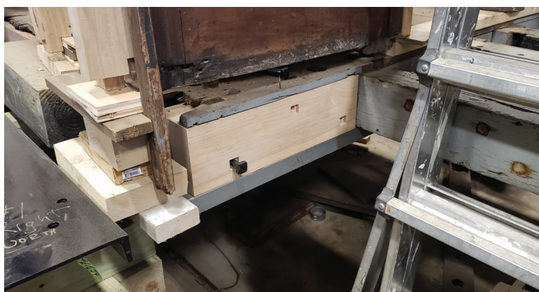
New precision cut pieces are spliced into the Narcissus platform. KO
