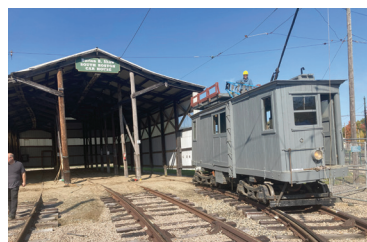
Trolley wire removal before demolition. TG
