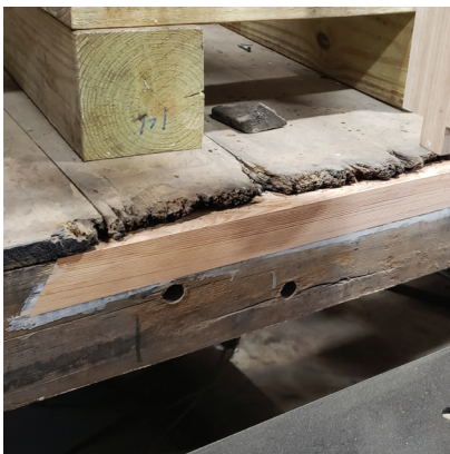
Above and Left: More precision-cut patches in the Narcissus frame fabricated by master woodworker Seth Reed. PM
