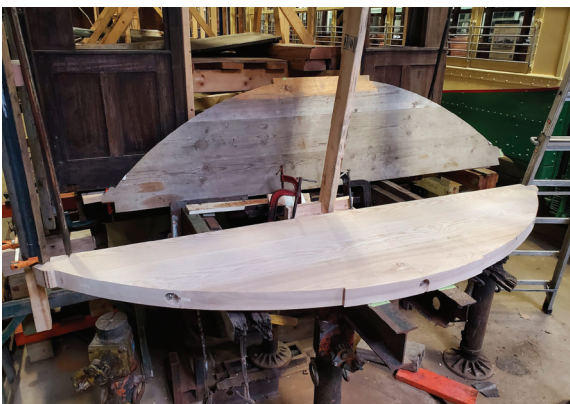
Left: Newly fabricated crown pieces will form the cab floors at each end of the car.
