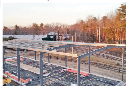
Erection of framing advances in early December.
