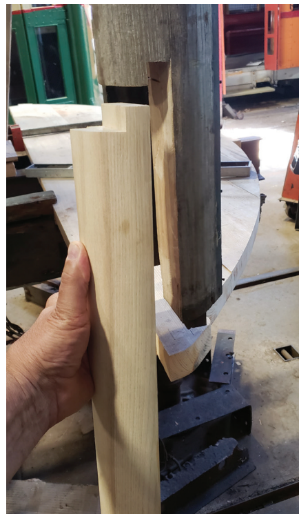
Above and Left: More precision-cut patches in the Narcissus frame fabricated by master woodworker Seth Reed. PM
