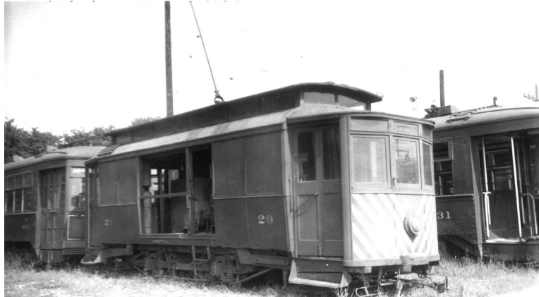
#29 built by St. Louis Car Co. (1899) on a design by Ford, Bacon & Davis. Converted to a rail grinder and then sand car. Ultimately restored in its sand car configuration and is still operated from time to time by the successor transit agency.
