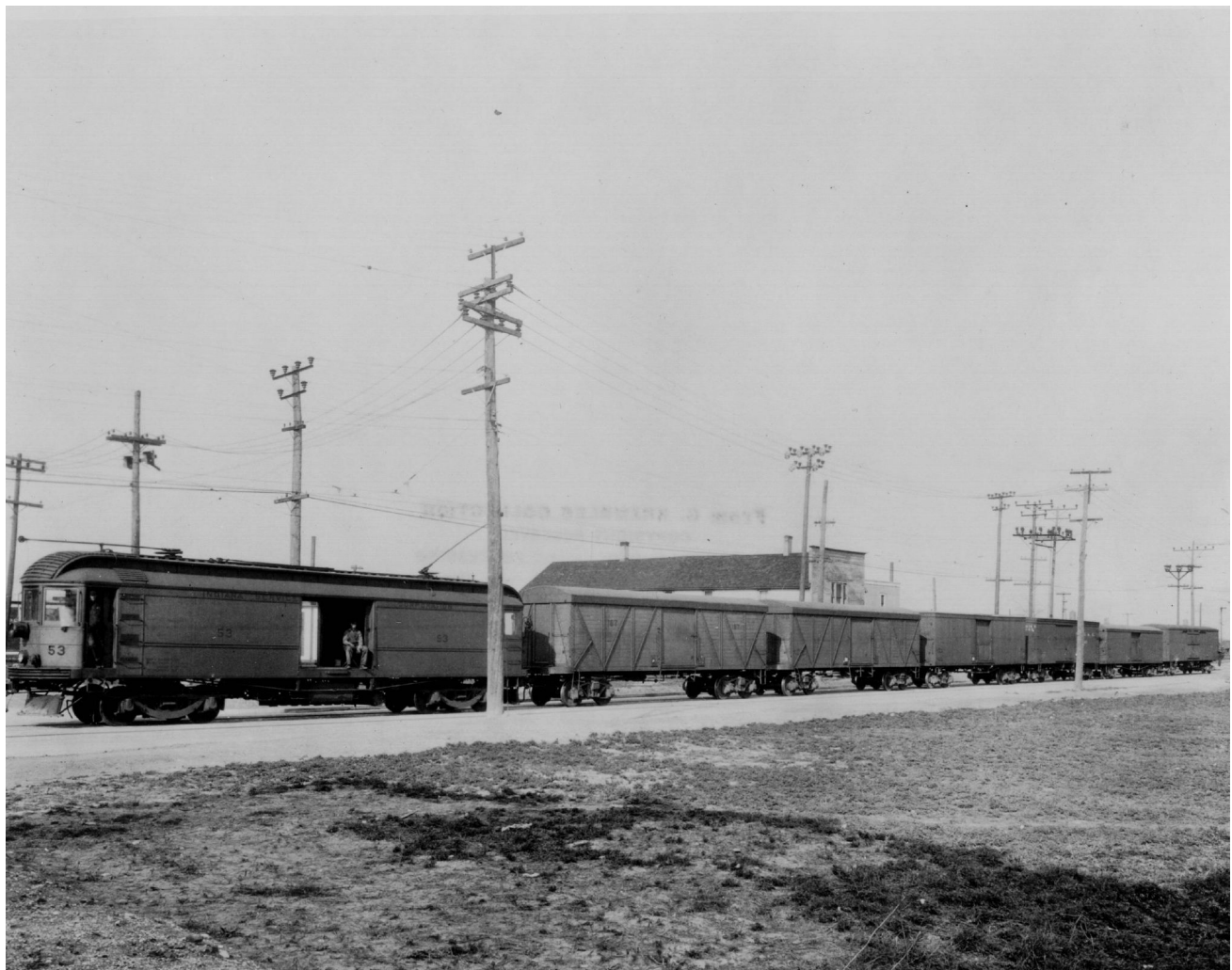
Freight motor No.#53 - rebuilt c. 1913 in company shops from wrecked passenger car
