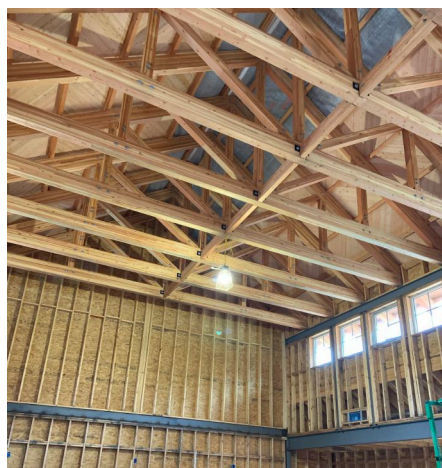
Framing and roof structure from main floor.
