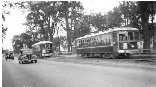
No. #60, 31 ft. safety car - JG Brill (1922) acquired 1931 passing No. 50, 33 ft. closed car - Kuhlman (1918) in Waterville
