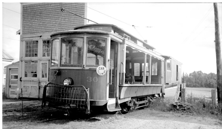
#30, built by Brill, after conversion to a sand car from a second-hand closed car obtained from an adjacent railway in 1927. The car is at the carhouse located in Oakland.
