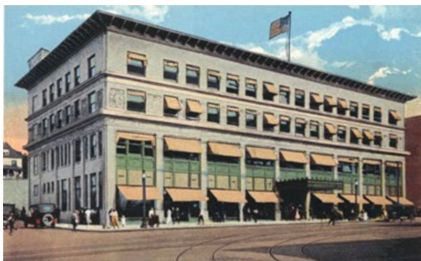
The line's new (1918) terminal in Akron. It included a double train shed containing eight tracks - some 32 interurban trains an hour arrived at or departed the terminal.
