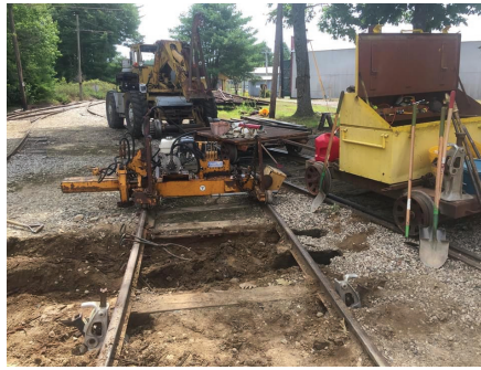
Above: Before the Shop switch project moved ahead several ties in the yard were replaced. PM
