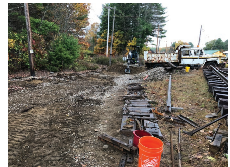
Above: A large dump truck is used to haul away gravel that was under the old switches. KO
