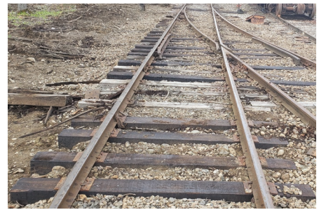
Above: The newly replaced ties are easily spotted by their dark creosote color. PM
