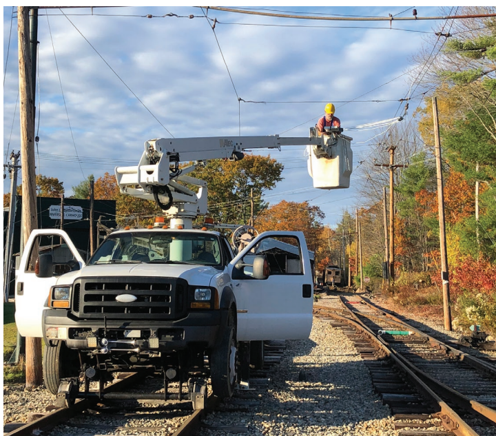
Left: Acquisition of this high rail bucket truck, enabled by a generous donation, greatly improves productivity of the overhead department as precise positioning is fast and easy. Here Overhead Superintendent Rob Drye adjusts wire over the north loop switch. KO
