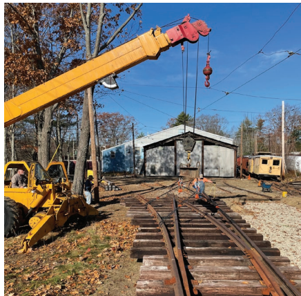
Above: The MK-36 crane is positioned to swing one of the new switches into place. JS
