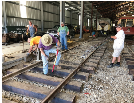
Above: Track crew members lay new track in the front extension of Fairview Car House. JS
