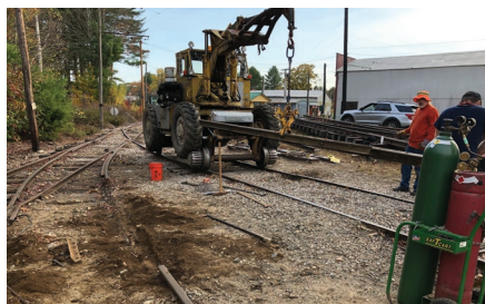
Above: The Pettibone Speedswing lifts and removes components of the old switches. JS
