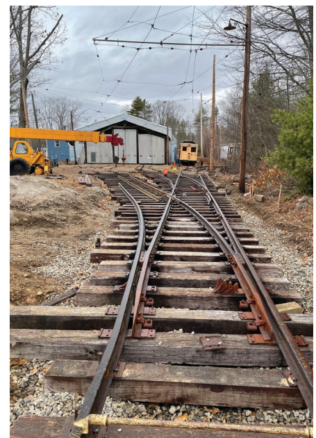
Above: The new switches as they appeared at year end. Work for spring 2021 includes installing switch stands plus final ballasting/tamping. JS
