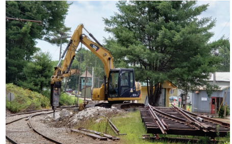
Above: As the in-ground work on the Shop switch project began, clearance around a rock outcropping was widened by this machine. Note the pre-assembled switch at the lower right. PM
