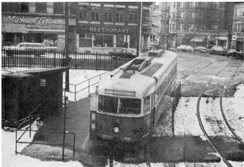
Number 3327 at Broadway and Tremont Street — February 2, 1962
