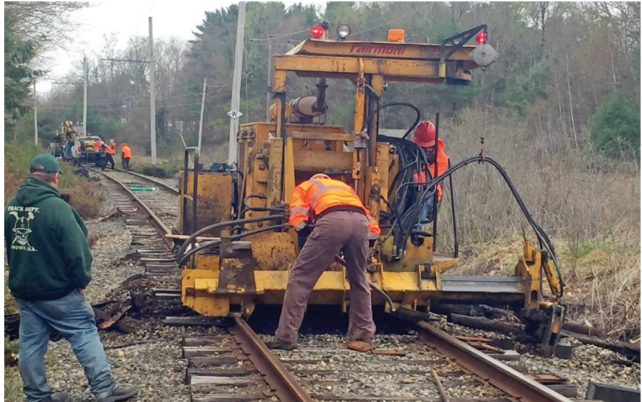
Above: Mechanized equipment can greatly accelerate track work. Here Maine Track Maintenance's tie inserter pushes a new tie between the stone ballast and the rail on which it sits, a task much more arduous if done manually as it has been by Seashore crews since the Museum's earliest days. JB
