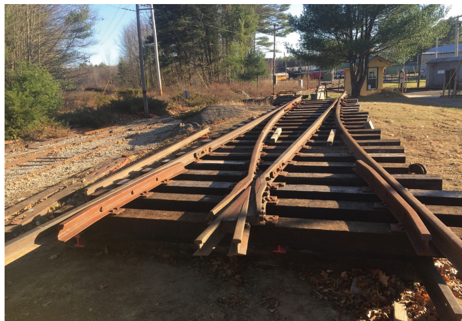
Above: The track crew has essentially completed assembly of a second brand new turnout to replace one of the very worn century-old ex-Sanford switches in the restoration shop yard. Plans for late 2020 call for removing and excavating the old switches then lifting the new ones in place JB
