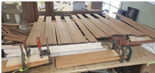
Left: Seth Reed removes many layers of finish coats to prepare one of The Narcissus ' doors for new finish. Above Top: The car has a seemingly endless supply of wood finish pieces, some requiring patching as well as refinishing. Above: An array of carefully stripped pieces each featuring inlays. In the foreground are pieces undergoing repairs. PM
