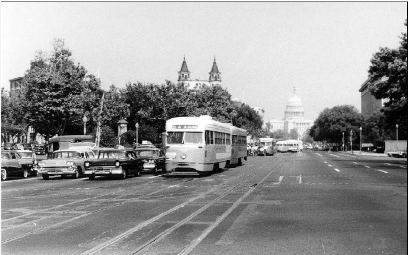
Below: About six years later, streetcars were still plentiful on Pennsylvania Avenue in Washington, D.C. The cars shown here, of the same type as the Museum's 1304, drew power from an underground conduit, as overhead trolley wires were prohibited in downtown Washington. Similar systems were used in New York, London, and Paris. Washington streetcars ran until 1962. RA
