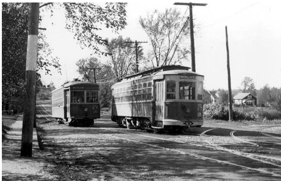
Above: Two Eastern Massachusetts Street Railway cars pass in Haverhill on Main Street in 1936, shortly before streetcar service ended. Seashore has cars very similar to both. The car on the left, of the 6000 series, is similar to Seashore's 7005 and the car on the right is of the same type as 4175. CD
