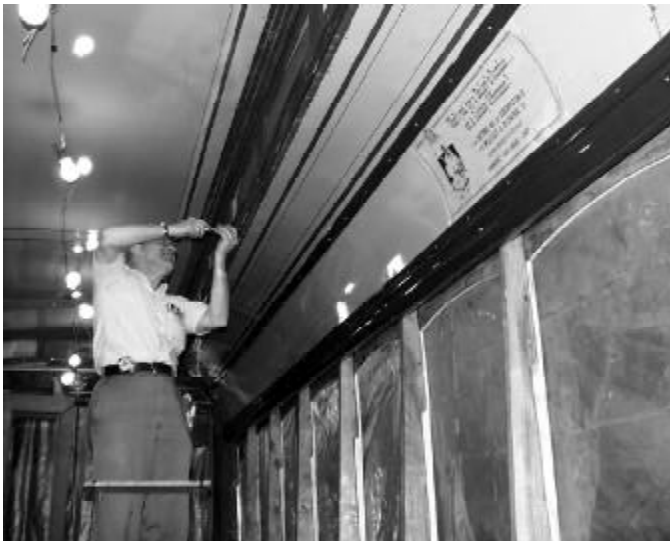
Below: Bob Reich installs some of the newly refinished interior woodwork in Bay State Street Railway No. 4175. The very careful and accurate restoration of this car is making steady progress as the glistening surfaces show. JS
