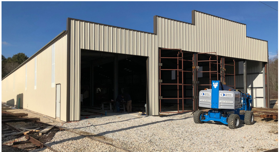
Two views of Fairview progress. Above: The steel framing for the 60-foot front extension has been erected and forms are in place for the concrete pad to be poured in the front corner. Below: At year end the exterior sheathing is all in place. A roll up door will fill the left bus and streetcar opening and framing for swinging doors is being fabricated and installed for all four of the main storage tracks. JS
