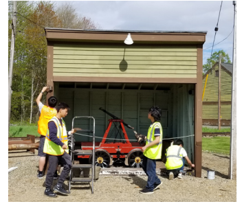
Above: Volunteers painting Arundel Station. Plans are being made to offer visitors paid rides on the hand pump car starting in 2019. PM
