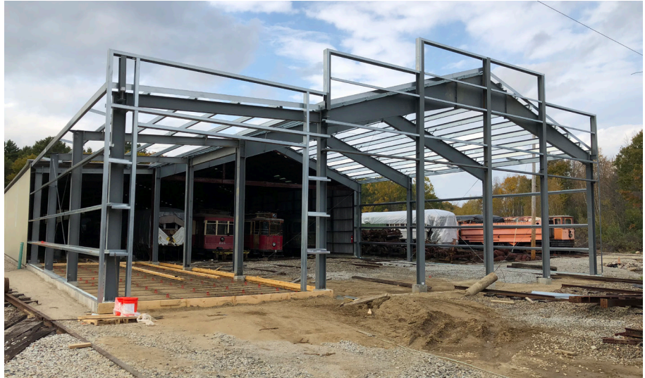
Two views of Fairview progress. Above: The steel framing for the 60-foot front extension has been erected and forms are in place for the concrete pad to be poured in the front corner. Below: At year end the exterior sheathing is all in place. A roll up door will fill the left bus and streetcar opening and framing for swinging doors is being fabricated and installed for all four of the main storage tracks. JS
