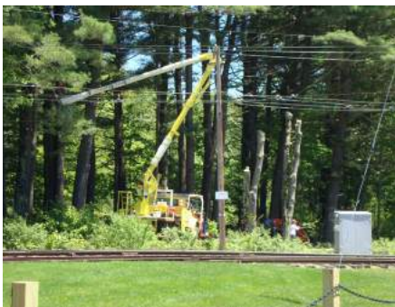
Below: Tree work, including harvesting salable lumber and trimming branches encroaching on infrastructure, was a significant project this year. PM
