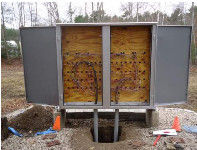
Below: A view of the surprisingly intricate wiring that controls the wayside signals that are designed to prevent accidents between operating cars. CB
