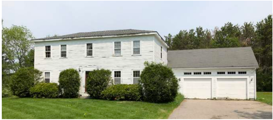
Above: The house adjacent to the Museum entrance, which was purchased with member donations, from the Butler family some years ago has, until recently, been rented to outside tenants. This year the Board voted to adapt the house for use by the Seashore Library giving much needed work space. JS
