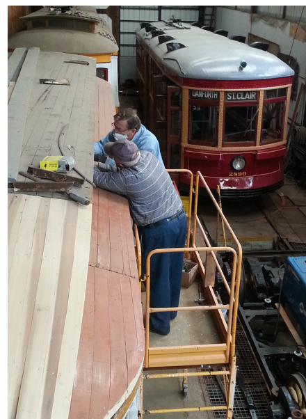
Above: Lexington and Boston No. 41 on its temporary wood-framed truck enabling it to move out of the shop during the shop roof project. Right: Volunteers Dick Avy and Jim Mackell work on the car's clerestory windows. In the background is Toronto Peter Witt No. 2890. DJ
