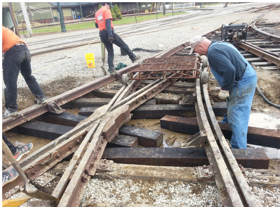
Below: Members of the Museum's track crew replace deteriorated ties under one of the switches in the yard serving the Burton B. Shaw South Boston Carhouse. These same rails served City Point Carhouse in South Boston until its closure in 1953. Volunteers then relocated the track fan to Maine. JS
