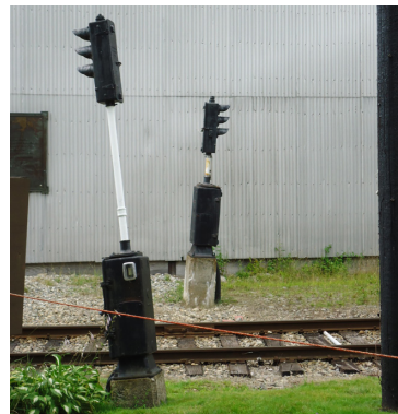
Three views of signal work near Morrison Hill Station. Upper: Before an after shots of signals that received new, more stable concrete bases. Below: Morrison Hill Station with both main line and crossing signals. CB
