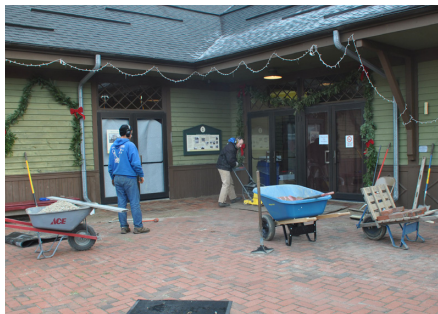
Above: Contractors smooth bricks at the Visitors Center platform to reduce tripping hazards. TS
