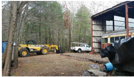
Above: Clearing and grading along Fairview Carhouse have prepared the area for column foundation repairs and for planned expansion to accommodate two rows of vehicles on this side. TS
