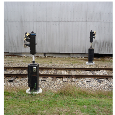
Three views of signal work near Morrison Hill Station. Upper: Before an after shots of signals that received new, more stable concrete bases. Below: Morrison Hill Station with both main line and crossing signals. CB
