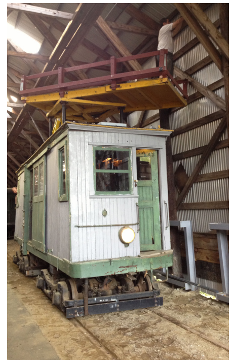
Above: Working from Claremont (NH) line car 4, Chris Randall installs Internet cables along the top edge of the interior wall in Highwood Carhouse. The wiring will support interactive kiosks and security systems. JS
