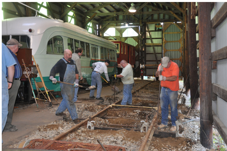
Above: Members of Seashore's track crew undertake the arduous job of replacing deteriorated ties inside Riverside Carhouse. Clearance for sliding the eight foot long ties under the rail is quite limited. DC
