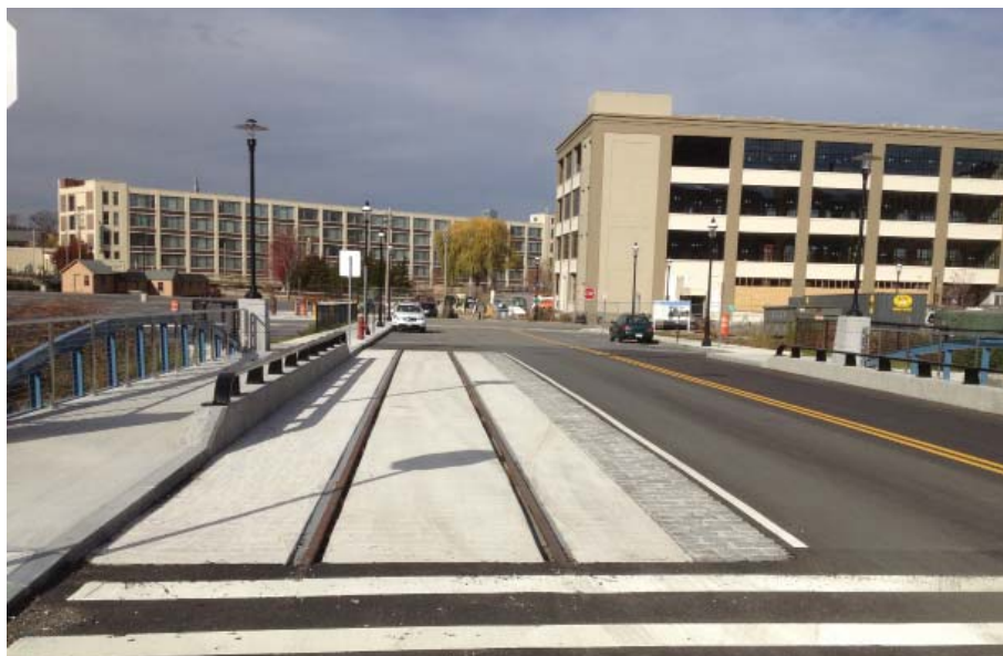
Above: A harbinger of things to come. A new bridge on Revere Street over the Hamilton Canal has rails installed in it in anticipation of the future line connecting to the Lowell train station. JS
