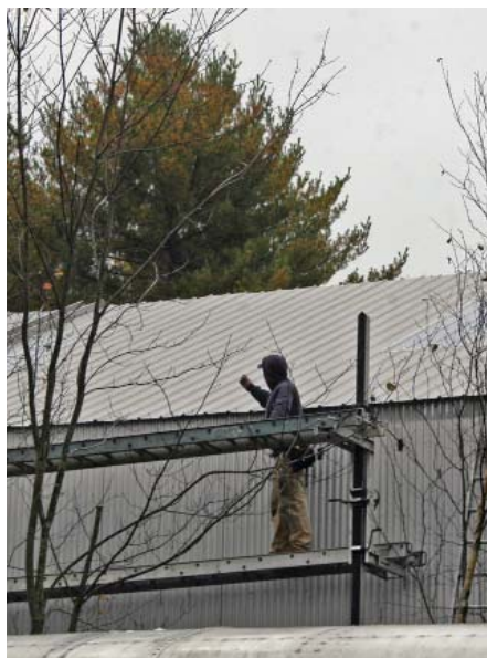
Above: A contractor adjusts staging used to install Highwood Carhouse's new roof. JS
