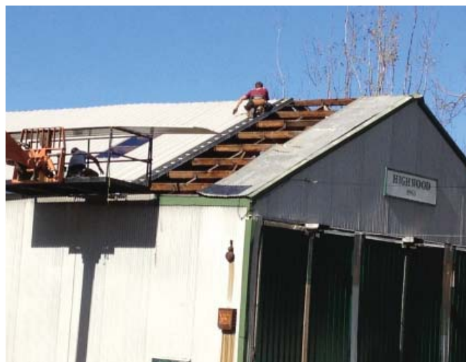
Below: A contractor's crew places new roof sheathing on Highwood Carhouse, a project made possible by a generous benefactor.
