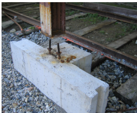
Above: A new footing in Fairview Carhouse after the main pour has been completed and stone backfilled. A second pour will fill the gap to the bottom of the column. The side slots are to support the frost wall running between footings. TS
