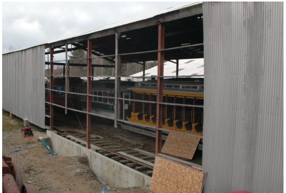
Below: New footings have been poured and the first sections of a frost wall between the footings at each column have been constructed. Future plans call for frost wall around the entire perimeter. TS
