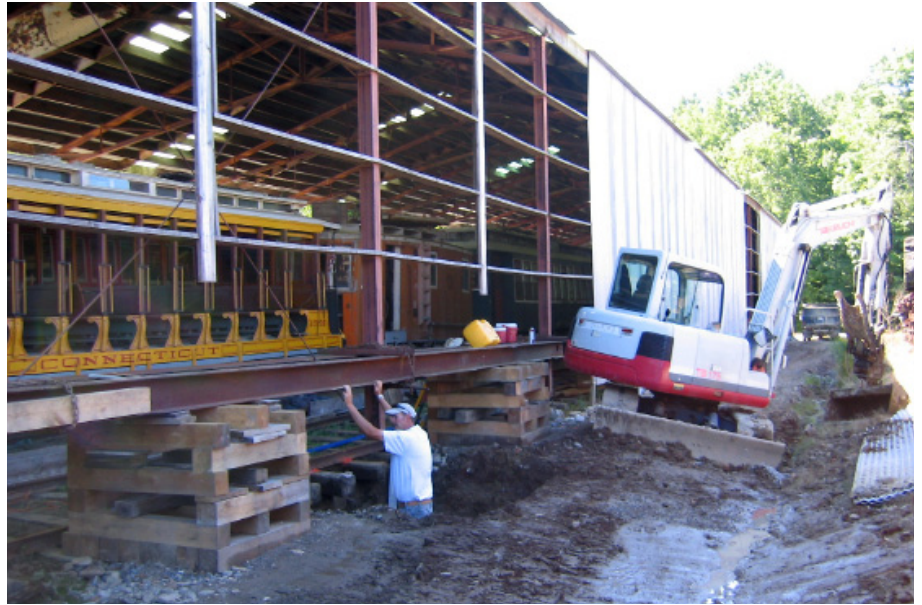
Above: Soil conditions around Fairview were a challenge to the contractor doing repair work. Considerable grading was required for equipment to reach the deteriorated footings. Here temporary blocking piles and beams support columns while new footings are excavated then have concrete poured. TS
