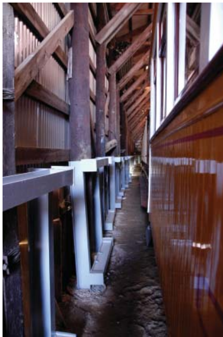
Above: Repairs to Highwood Barn consisted of heavy steel beams set in concrete to reinforce the bases of deteriorated original wooden poles. JS
