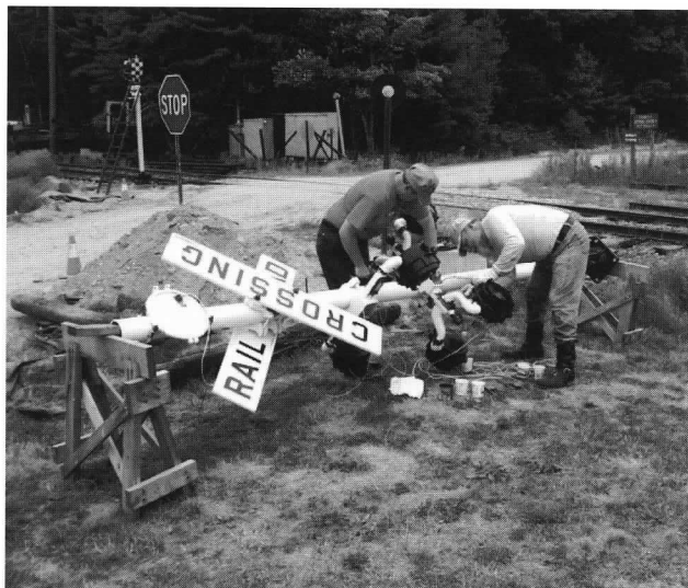
Above: David Shaw and Chet Bishop renovate the crossing signal that protects the McKay Boulevard main line crossing behind the shop. JS Below right: In a photo that could have been taken nearly 100 years earlier, Connecticut open delivers a crowd to a summertime event. JS Below: A crew places a truck for Philadelphia PCC 2709 on the track after repairing a damaged motor. The car was soon running again. JS
