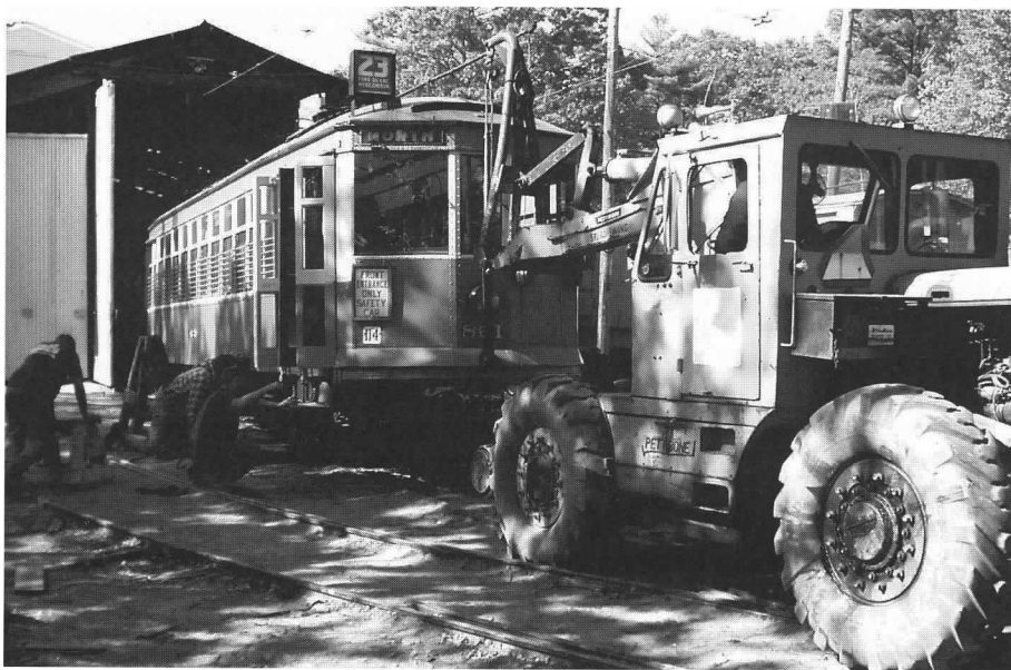
Above: Milwaukee 861 has had most of its underfloor wiring replaced as part of its gradual mechanical upgrading. Here a Pettibone tractor is used to lower the body back onto one of its trucks. JS
