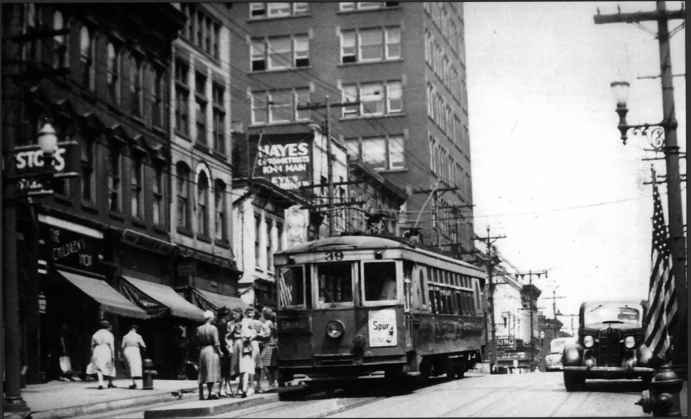
Above: This shot in downtown Wheeling, West Virginia shows Seashore's curved-side No. 39 pulling up to a loading platform on Main Street on a warm summer's day in 1945. The restoration of this car continued in 1998, making progress toward the day when the Museum will be able to recreate the riding experience that the women waiting to board the car would enjoy a half-century ago in wartime Wheeling. WG
