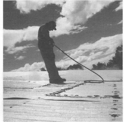
Above and Left: Conrad Misk and Amy Litchfield undertake the project of refastening and sealing the shop roof, to reduce the number of leaks inside on rainy days. DC/FM
