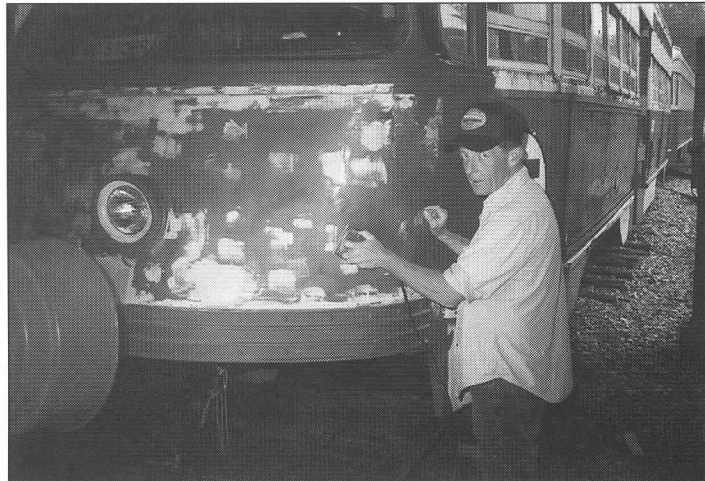
In another volunteer PCC restoration project, Peter Folger uses a power sander on the dash of Boston All-Electric car 3221. FM
