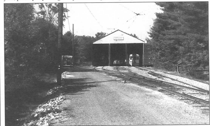
Below: The road leading to Highwood Carhouse was widened and extended this year, plus rip-rap lining was placed along the edge to prevent erosion. JS
