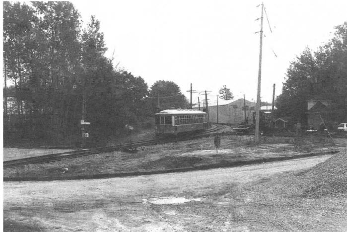
This area, now known as McKay Commons, received extensive attention during the year as many tons of rail, structural steel, track material, and other items was removed to less visible storage. Landscaping will follow in 1994. In this view, Milwaukee 861 passes on the main line in the background. JS
