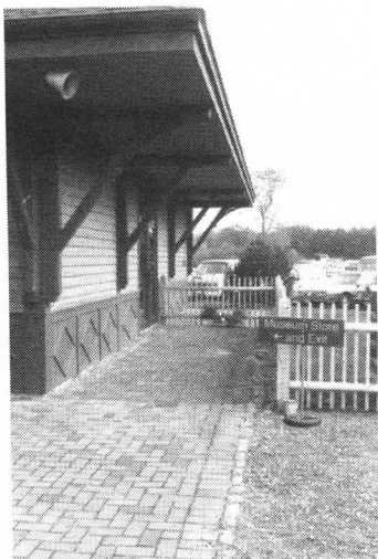
This new brick path at the south end of the Visitors Center is used by exiting visitors, taking them through the Museum Store on their way out. JS
