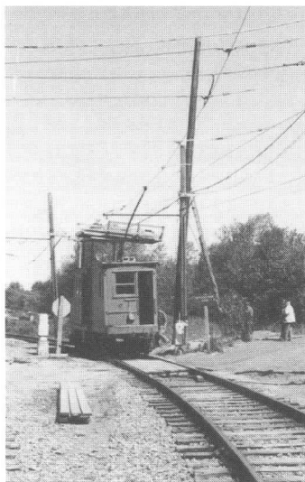
Overhead wire maintenance tasks undertaken by volunteers during the year included replacing a broken pole at Riverside using ex-Claremont (NH) line car No. 4. PC
