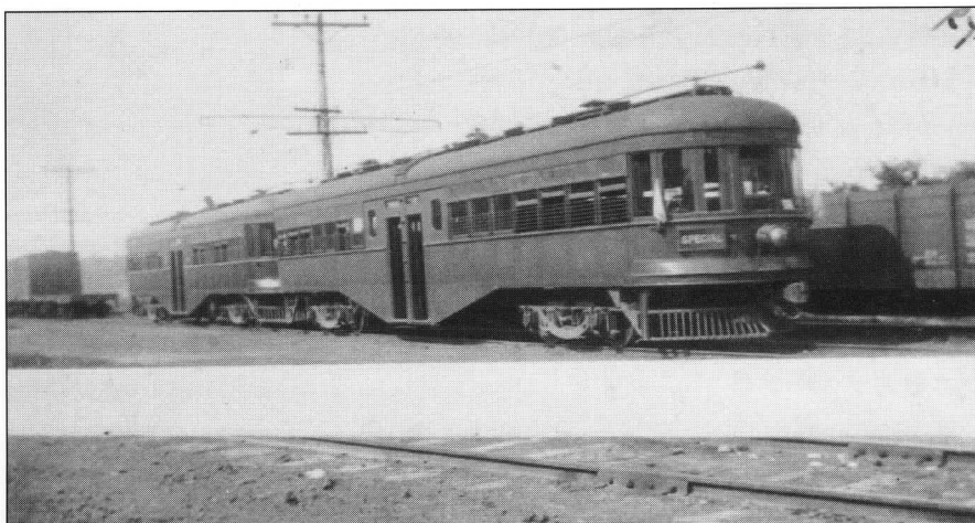
KANSAS CITY, CLAY COUNTY & ST. JOSEPH RAILWAY: This view, taken in 1926, shows No. 25 (sister to Seashore's No. 24) operating as part of a two car train. The cars weighed 85,000 pounds and were capable of 75 miles per hour.
