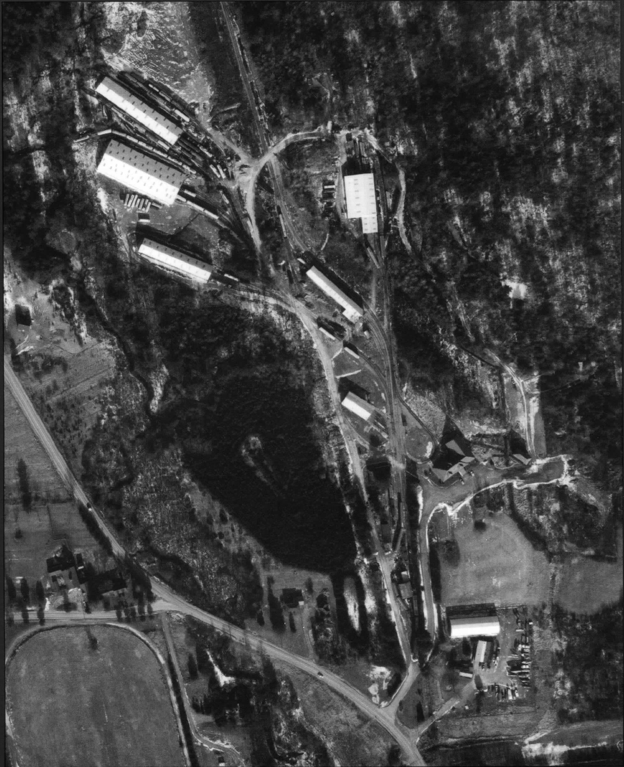
This enlargement of one of the aerial photographs used for topographical mapping shows the main Museum site. The land purchased from John Smith in 1991 is at the lower right hand corner, extending below the visitors center, surrounding the boat yard, and extending off the right edge of the photograph.
