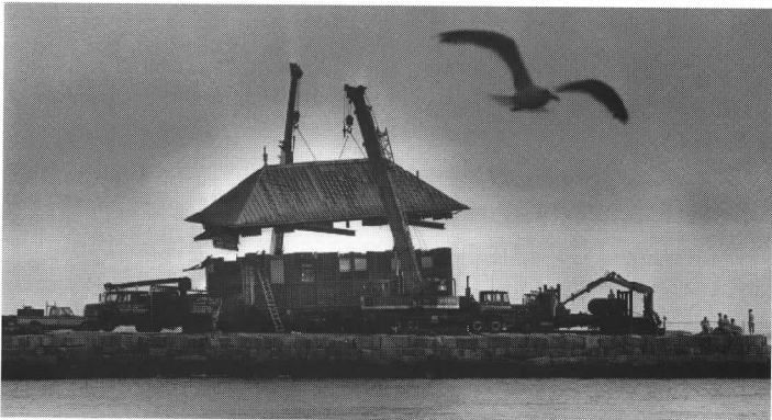
These press photos recorded Northampton's progress: Above: The roof is raised to clear the body which then will be driven ahead so that the roof can be lowered onto transport dollies. Below: The roof and body proceed in convoy along Ocean Ave. about 7:00 am.
