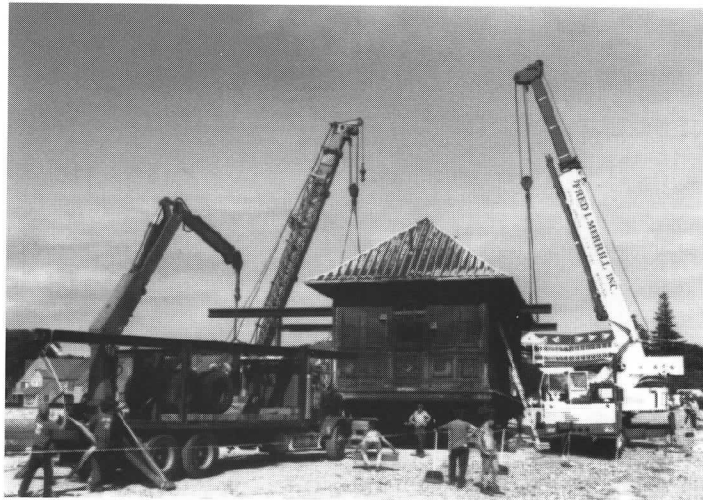
Below: With the Colony Hotel visible in the background, two cranes and the building movers prepare to lift the roof from Northampton.
