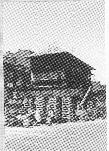
ABOVE: After the crane debacle, the contractor engaged Payne Building Movers to lower the station with jacks. B. CLARKE
