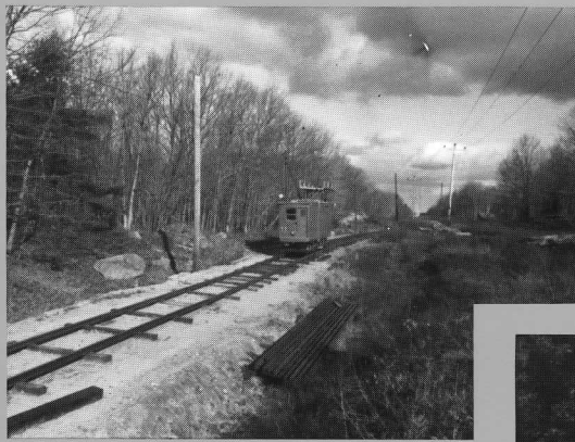
The first electric car over the skeleton track is Claremont, N.H. line car No. 4, used to string trolley wire. F. PERRY
