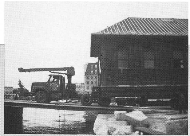
ABOVE: Northampton was loaded over a ramp of eighteen 12 by 12 inch steel beams, spanning nearly 30 feet of open water. P. CALCATERRA
