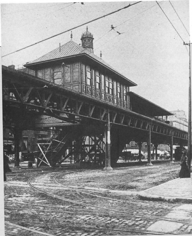
ABOVE: Northampton nears completion in 1901, one of ten identical El stations. F. CHENEY COLLECTION
