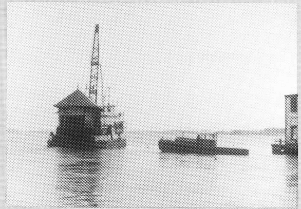
ABOVE: The elevated station heads to sea after the loading was completed successfully. P. CALCATERRA
