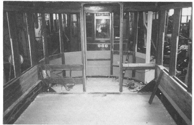
TOP: The front platform structure of Twin Cities 1267 after renewal and rebuilding of steel frame members.
