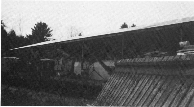
Carbarn work completed in 1988 included application of roof sheets to the rear extension of Fairview Barn, providing covered space for eight more cars.
