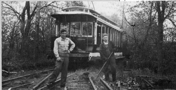
Track construction during very early Seashore days. Ted poses with long-time member and caretaker Joe McLaughlin and B&S 31 near the current site of Shop 1.
