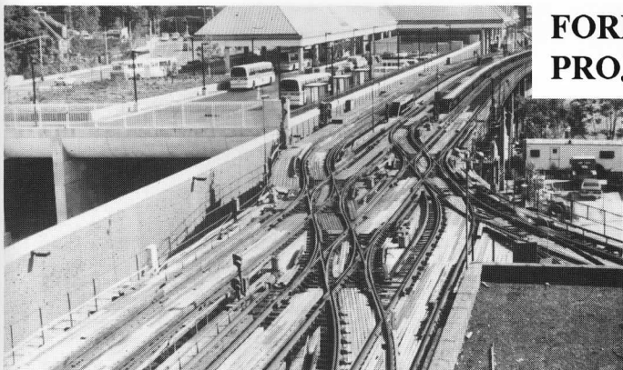
A view from the Tower reveals three double-slip switches. The new Forest Hills Station is visible in the background. TSdeB
