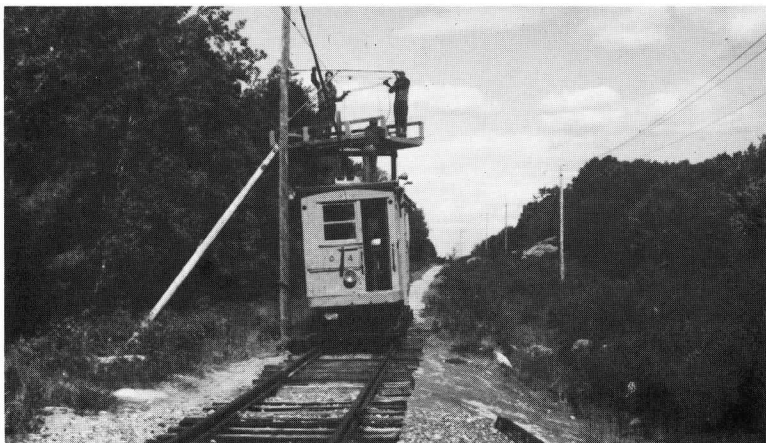
Claremont, N.H. line car No. 4, still in MBTA yellow from its lease to that agency, is used to center the overhead at the end of the Museum's main line. TSdeB
