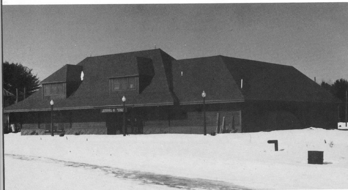
The museum's Visitors Center is an imposing structure even on crisp winter's day. Gradual progress at installing heating and insulation inside bring nearer the day when this will be a true year-round facility. TSDeB
