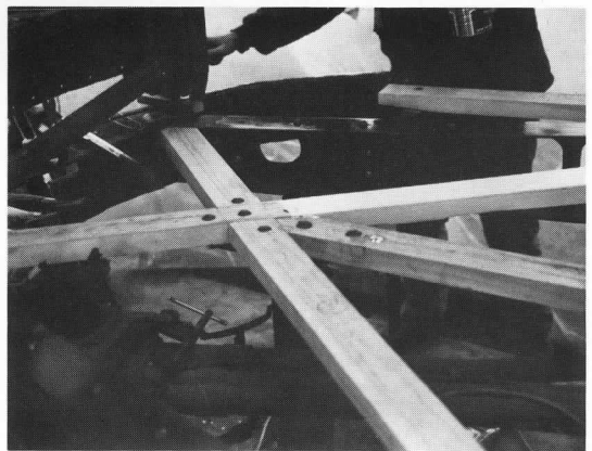
Here the new platform knees are in place on 4175 and new "X" bracing has been fit carefully in between. The next step will be installation of flooring. TSdeB
