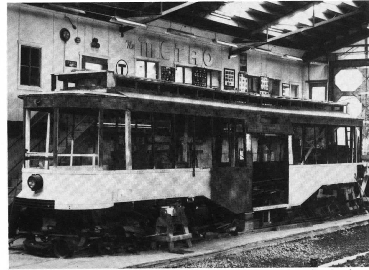
Center Entrance car 6131 with lower steel work in prime and new side roof section that has been replaced. TSDeB
