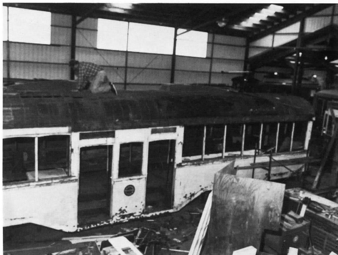
4. Cleveland Railway 1227 while having all new sash, doors and roof sheathing manufactured, was found to require more than anticipated underframe work at a later period. Temporary steel plates were welded to the carbody to reinforce car during the interim period.
