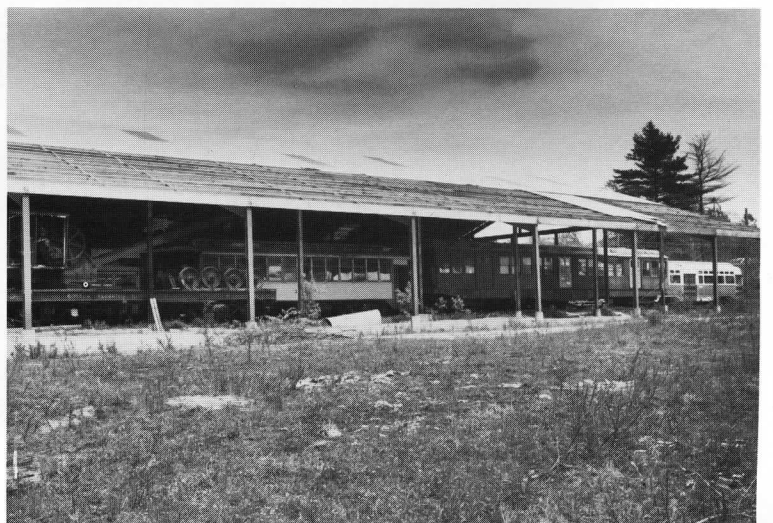
5. Construction of the south lean-to on Central Barn was well along at end of 1985, with much more protection being afforded to rolling stock already stored in main part of structure.
