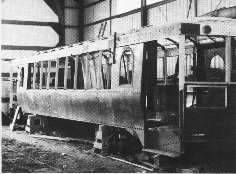
Wheeling curved side Car 39 shown in its present state of reconstruction, and in readiness for resheathing of the roof. Much of the work done during the winter months had consisted of glazing the window sash, work that won't show results until reassembled on the car at some distant point in the future. When 39 has been completed only approximately ten percent of the original car will be left. As an example little of the original steelwork will be left, the bolsters and bumpers being the few remaining salvageable steel items. Richard M. Wagner's publication "Curved-Side Cars Built By Cincinnati Car Company" has been a valuable aid in reconstruction of this car. 39, will be one of the few survivors of the entire group shown in this book. TSDeB
