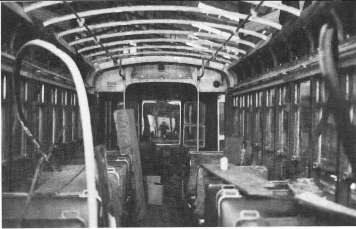
ABOVE — Extensive deterioration of the central section of Third Ave. 631's roof, constructed of hardboard (Masonite) covered with canvas necessitated its removal and rebuilding from carlines up. TSdeB
