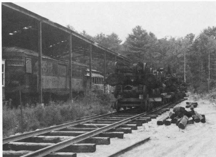
New truck storage track alongside Fairview Barn.
