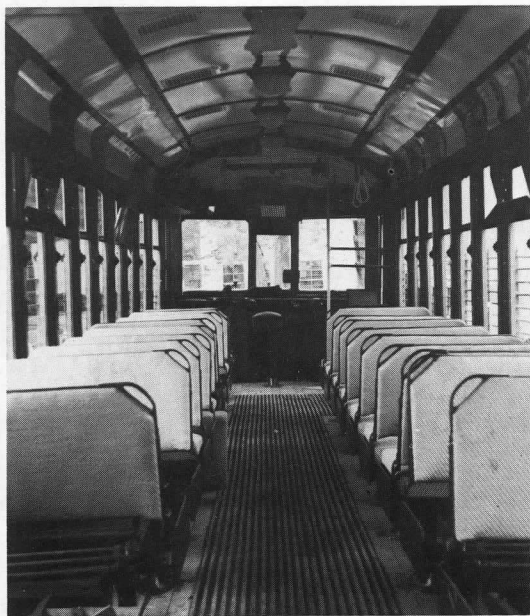
Rehabilitation of 861's interior was a major job requiring as it did structural repairs and re-engineering of the central part of the roof to prevent re-occurrence of the roof sagging. Also called for was replacement of headlining, re-installation of light fixtures, restoration of interior woodwork to varnished natural finish, and rebuilding and re-upholstering many of the cane seat cushions. MUNROE
