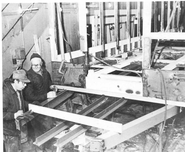
Donald Curry and Don Gawthrop busily engaged in the reassembly of 4547 that is going rapidly — This gives promise of this car's finally becoming operational again and restored to its appearance of many years ago, although the prospects of its ever running over the Brooklyn Bridge again seem rather slim.
