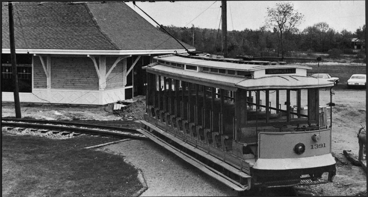
A closeup study of the Visitors Center, still in prime coat, reveals the detail of the paneling of the lower wall and of the roof braces salvaged from the old Boston & Maine Railroad's depot at Marblehead, Mass. Inspiration for the general outline of the building came from Canadian Pacific designs while much of the detail was copied from nearby Tower "C". Wooden poles with back guys are currently being replaced with more formal looking steel poles set in concrete with ornamental bracket arms and caps. — Woolnough —
