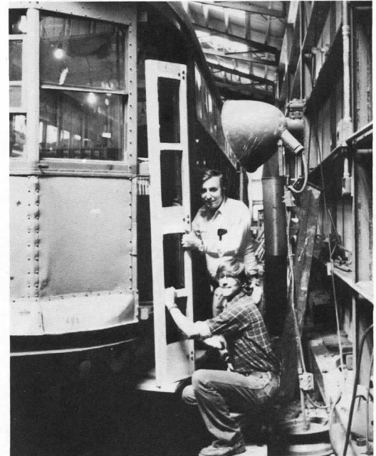
Father and son team installs the first set of new hardwood doors on 5821. The best of the old door sections were hastily refurbished to outfit Type 5, No. 5734, for its return to Boston to participate in the Riverside Line's 20th anniversary celebration. Lane Photo
