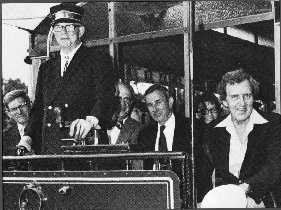
On the front platform of Biddeford & Saco No. 31 are, from left, State Rep. George Carroll, Foster Leavitt (at the controls), Alexander Hamilton, Theodore Santarelli de Brasch and Sen. Muskie being given, along with other guests and dignitaries, an inspection trip of the museum following the ground breaking ceremony. Woolnough Photo
