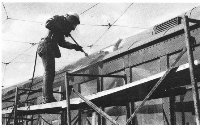
Cambridge Tunnel 0719 has roof sandblasted in preparation for repainting. — Lane
