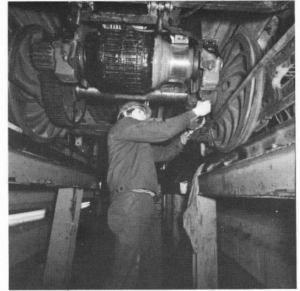
Rebuilt motor being installed in Line car S-71. — Brillante
