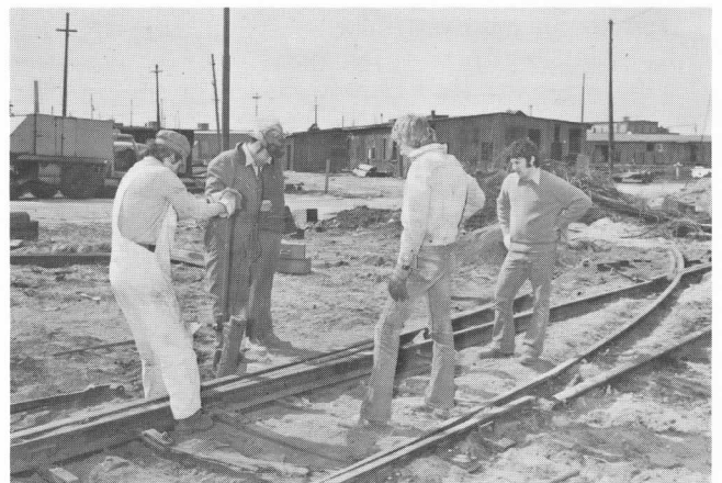
At the MBTA's Charlestown Yard, a group of volunteer members are engaged in disassembling a switch for removal. Brillante photo.
