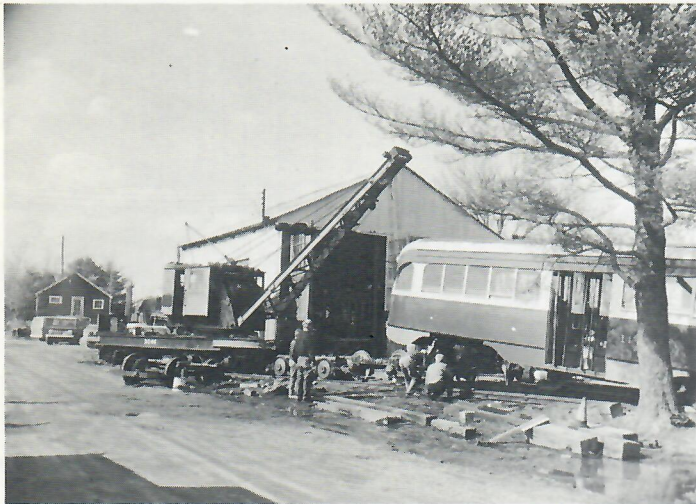
Pittsburgh P.C.C. car #1440 in process of being retrucked after standard gauging at Seashore, Washington, D.C. Standard gauge wheel and axle sets and housings were made available by MBTA for conversion. Brake rigging and track brakes were regauged on property. Our first P.C.C. should enter service in 1970. Photo by Gerald O. Boothby
