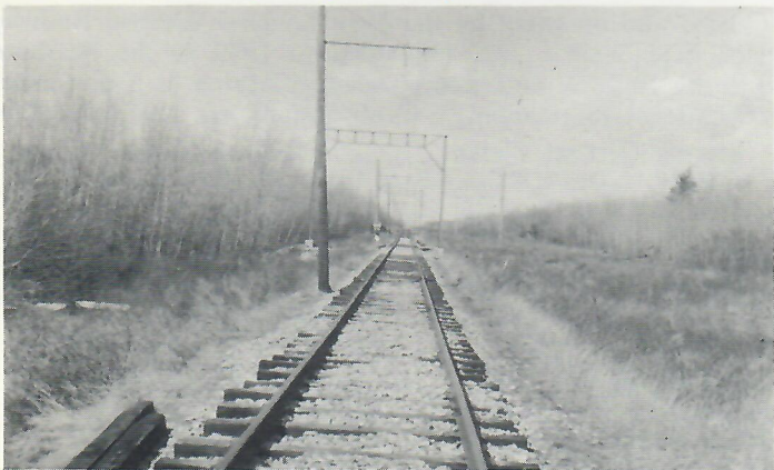
Looking North on Main Line showing recently ballasted and aligned track.
