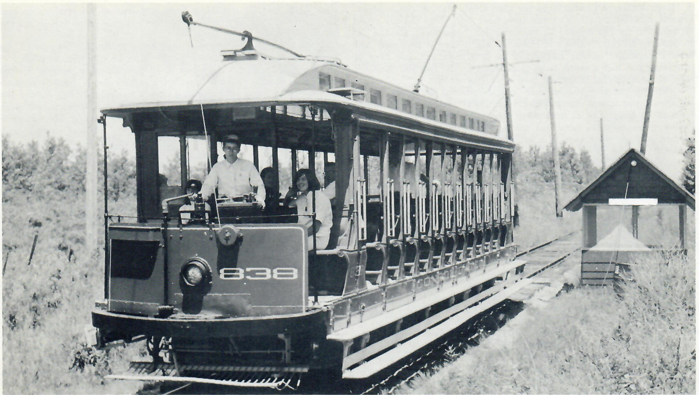
#838, 15-bench open built by Jones Car Co., poses at end of passenger run on a quiet summer's day. This ex-Connecticut Co. car continues to be one of the mainstays of the Society's passenger fleet since it went into service for us in 1957. Trustee Cecilia Clapp is shown at controls. Photo by Ernest A. Barstow
