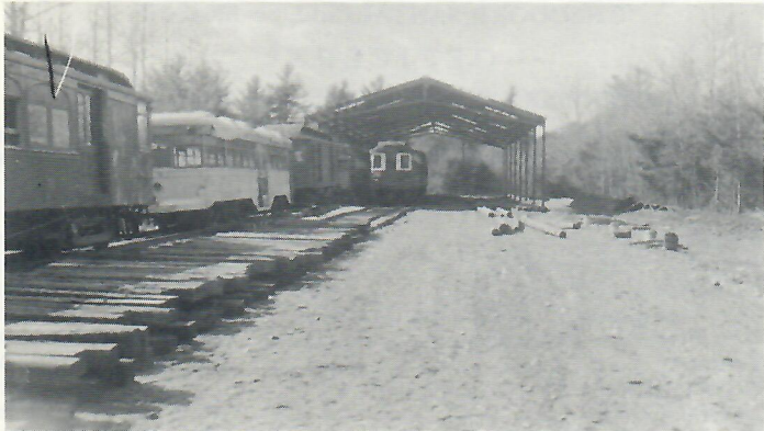
View of Central Barn with yard tracks 1 and 2 completed. Note ties set out on track 2 for completion of remaining tracks in 1970. Both photos Gerald Boothby
