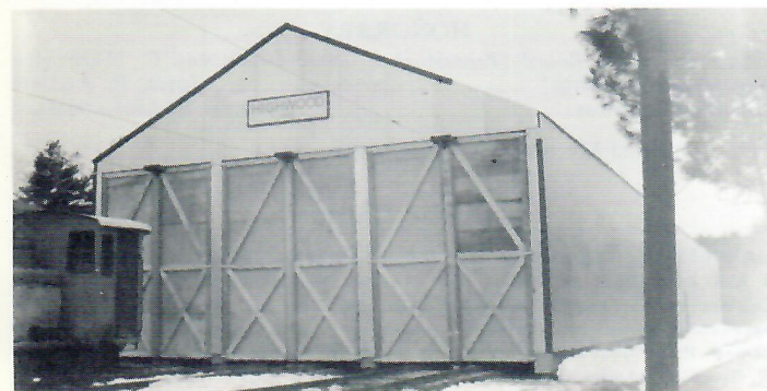
#4 Highwood barn, now virtually complete, awaits only coming of warmer weather, when doors will be painted and project completed. (Clapp photo)
