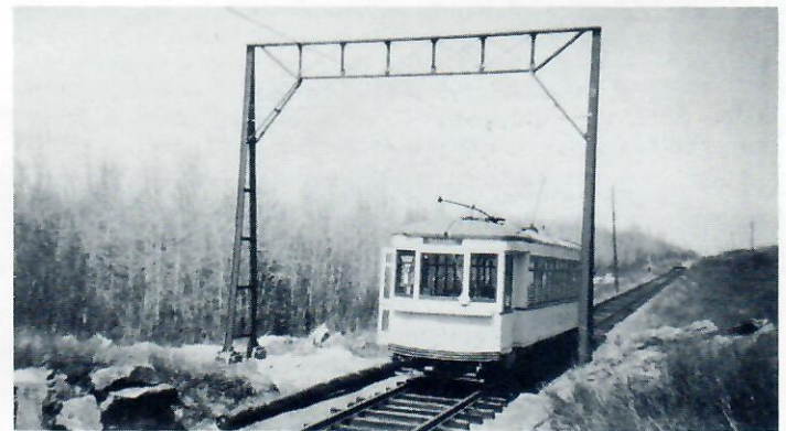
Looking North at tower #1 — Montreal 2052 ex Springfield, Mass. light weight poses. Track complete to tower site #3, Alexander Hamilton, 900' north. (John Coughlin photo)
