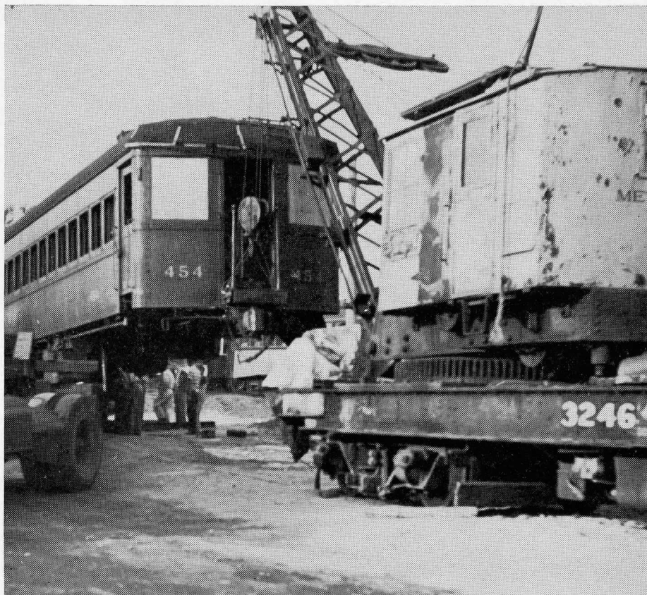
Sixty-two-foot car body is suspended by crane as Highway Monster is driven out and trucks placed before lowering. (F. J. Perry photo)
