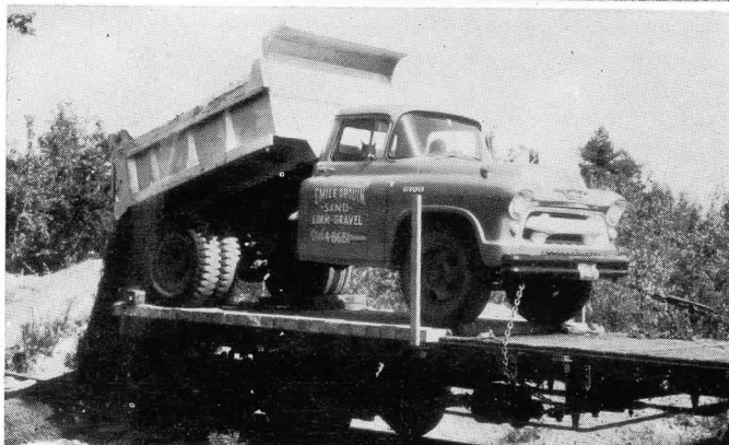
PIGGYBACK BALLASTING TECHNIQUE was used extensively in building the new line. (1) Truck drives on flatcar 0357 backed up to ramp. (2) Front of truck is chained down, locomotive 100 couples up. (3) Down the track. (4) Truck dumps as train moves along, spreading gravel in an even layer. (Doherty Photos)
