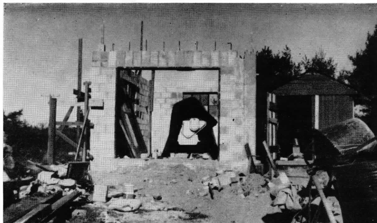
POWER STATION —Photo taken in Fall of 1951. Future expansion as required will be to the right. Main engine, under tarpaulin, has been cleaned and painted in readiness for car operation in 1952.
